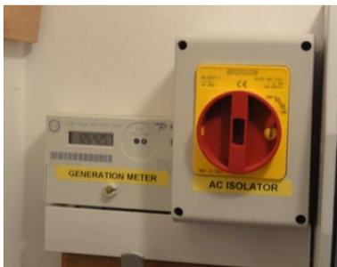
The inverter is fitted in the loft space with the generation meter located next to the consumer unit under the stairs. This had to be replaced at a cost of ca £350 with a modern one with circuit breakers instead of fuses.
